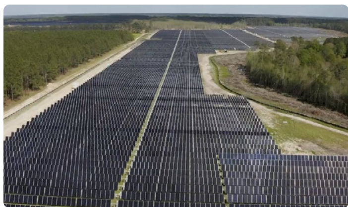
Banc of California helped finance the Snipesville III Solar Project in Georgia, which will provide low-cost, clean energy for generations. The facility can power up to 18,000 homes a year.
